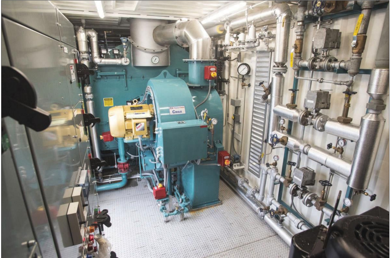
FIGURE 5. A 1,000-hp mobile boiler room shipping to a customer site for temporary steam supply.
