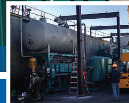
70,000 lb/hr Boiler and CataStak SCR System at California Dairies (top) and 150,000 lb/hr Mobile Deaerator at Roseburg Forest Products (right)
