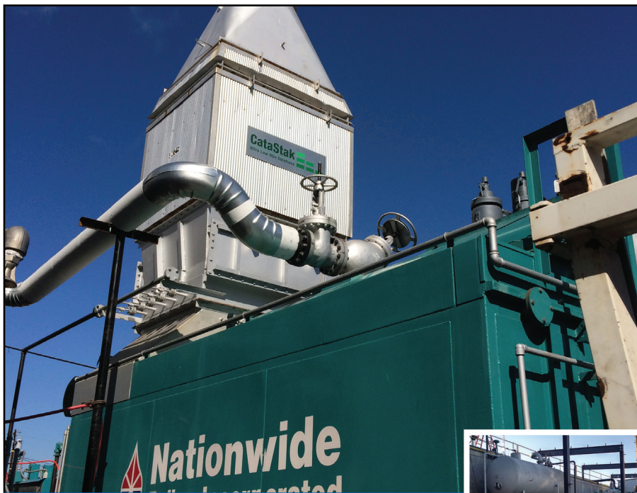
70,000 lb/hr Boiler and CataStak SCR System at California Dairies (top) and 150,000 lb/hr Mobile Deaerator at Roseburg Forest Products (right)
