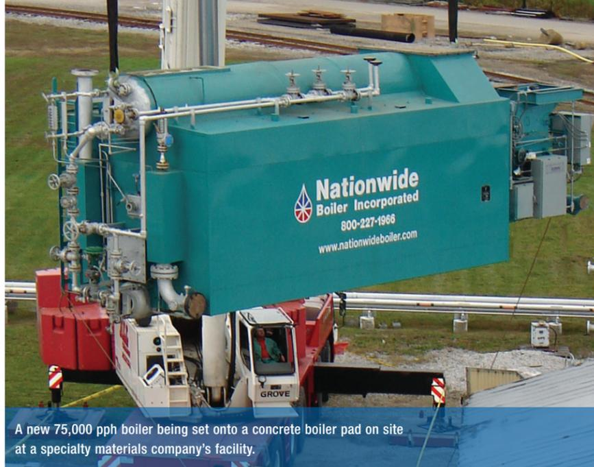
A new 75,000 pph boiler being set onto a concrete boiler pad on site at a specialty materials company's facility.
