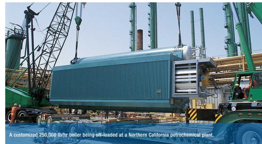
A customized 250,000 lb/hr boiler being off-loaded at a Northern California petrochemical plant.
