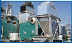
Nationwide Boiler provided two (2) E<sup>2</sup>Stak solutions, complete with two (2) new Babcock & Wilcox watertube boilers, CataStak™ SCR systems, EconoStak economizers and low NOx
