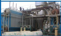
Nationwide Boiler retrofitted a 150,000 pph English watertube boiler with a CataStak™ SCR system and EconoStak economizer at Los Gatos Tomato in Huron, CA.
