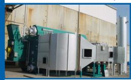
Nationwide Boiler supplied Del Monte, Modesto a new 50,000 pph Babcock & Wilcox watertube boiler with a low NOx burner, CataStak™ SCR system and EconoStak economizer.
