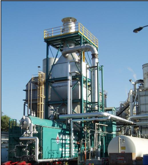
*A CataStak™ SCR system helped a paper mill in California reduce GHG emissions. The 120,000 lb/hr, 175 psi boiler operated at 5 ppm NOx and easily met local air quality requirements.*
