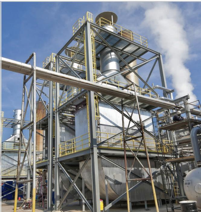
The multiple units were quickly installed and delivered by Nationwide Boiler within the quoted time-period and are currently in operation. Each unit was tested and exceeded the required NOx emission guarantees, performing at 3 ppm NOx and 2.5 NH<sub>3</sub> slip. In addition, installation of the new CataStak™ SCR system and EconoStak economizers provided boiler thermal efficiency gains of 2%, helping the customer to reduce fuel costs and increase efficiency.
