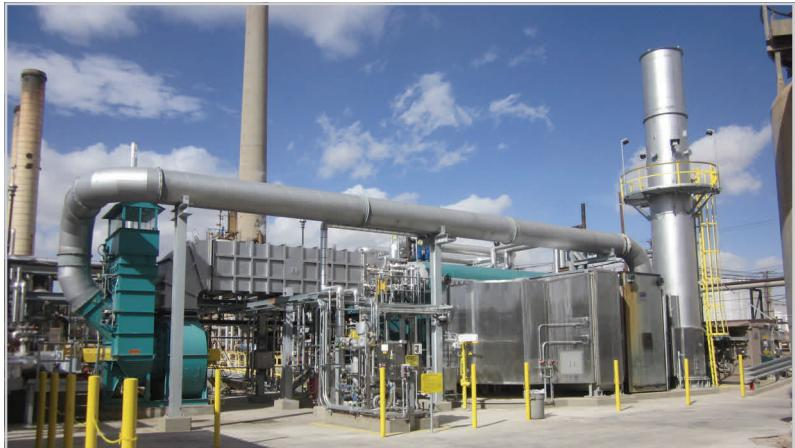
To meet NOx levels of 12 ppm (and future single digit NOx requirements), Nationwide Boiler also supplied a 19% Aqueous Ammonia CataStak™ SCR System with a vaporizer and 10,000 gallon aqueous ammonia storage tank with forwarding pumps, unloading station and controls.
