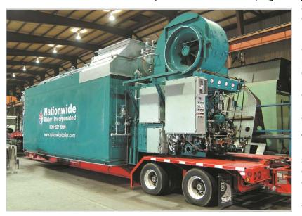
Following installation of the temporary boiler, the existing 90,000 lb/hr boiler was converted to burn natural gas. It was returned to service after the completion of the conversion program. Operation of the 40,000 lb/hr unit continued
