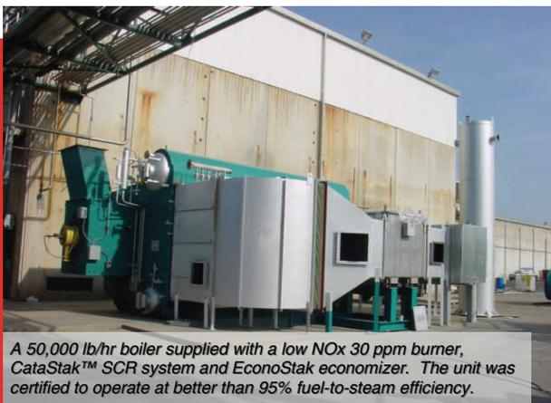
*A 50,000 lb/hr boiler supplied with a low NOx 30 ppm burner, CataStak™ SCR system and EconoStak economizer. The unit was certified to operate at better than 95% fuel-to-steam efficiency.*
