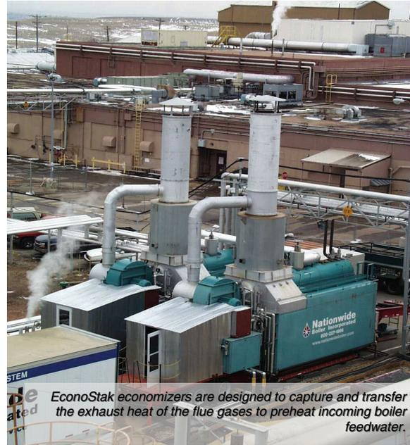
EconoStak economizers are designed to capture and transfer the exhaust heat of the flue gases to preheat incoming boiler feedwater.
