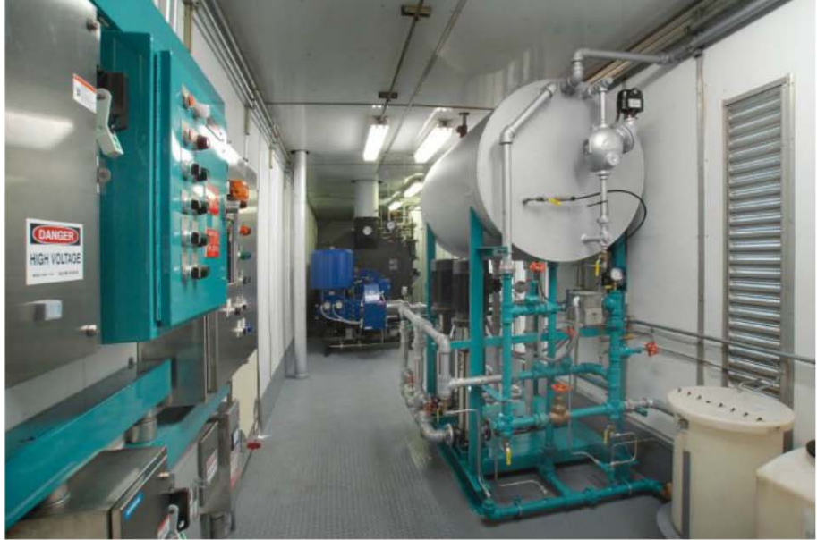
Mobile boiler rooms are enclosed-van units that include all the necessary auxiliary equipment for reliable steam production.
