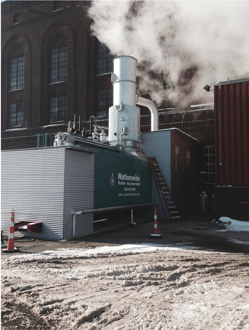
An 82,500 lb/hr trailer-mounted watertube rental boiler is equipped with front and rear enclosures.
