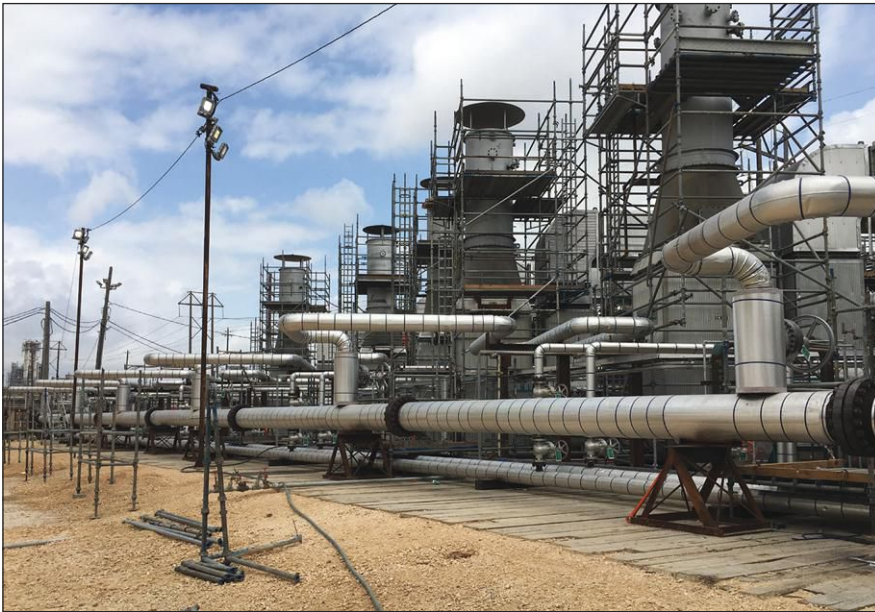
Figure 3: The temporary boiler equipment supplied process steam to meet facility demand for more than three years and was also instrumental in returning this facility to an operable state after the “Big Texas Freeze of 2021.”
