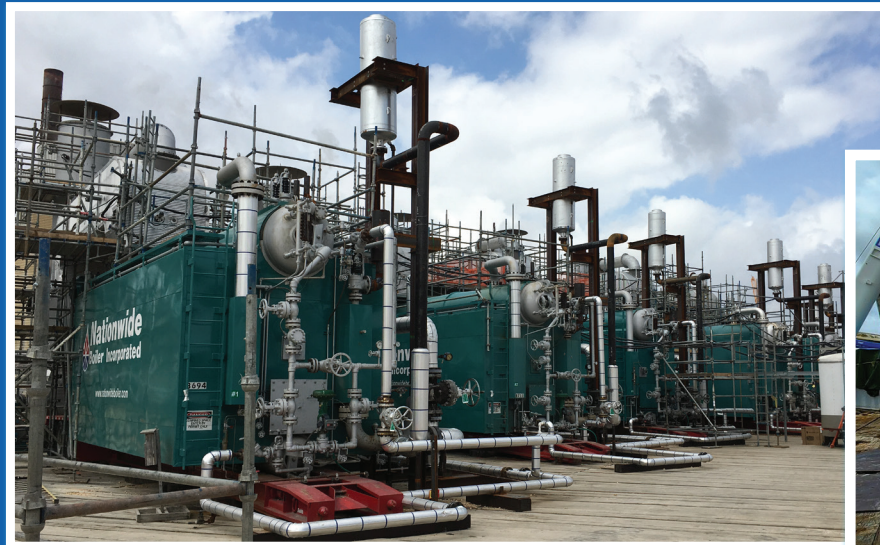
Installation of six (6) 75,000 lb/hr trailer-mounted boilers with SCR's (above)
