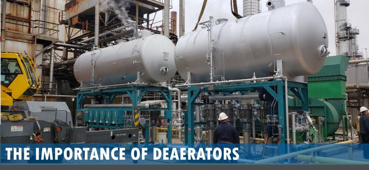
Deaeration of boiler feed water is primarily known to remove dissolved oxygen from the water, however, there are four additional advantages: (1) carbon dioxide removal, (2) improved operation, (3) improved heat transfer, and (4) energy savings.
