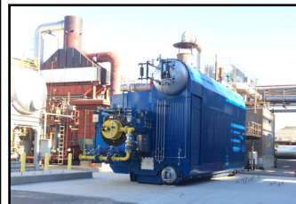
Installation of a 150,000 lb/hr Babcock & Wilcox Boiler, Sold by Nationwide Boiler to a California Food Processor
